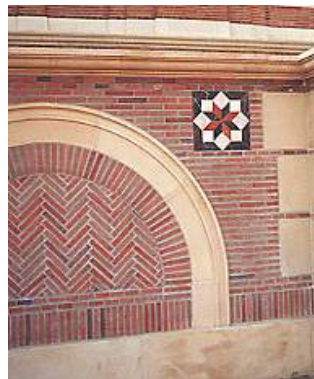
Brick and other masonry elements lend themselves to exquisite details. Blank walls should not be unarticulated, but have interest through coursing and materiality.
