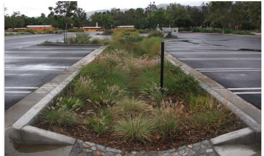
Bioswale installation, The Los Angeles Zoo, Los Angeles, California
