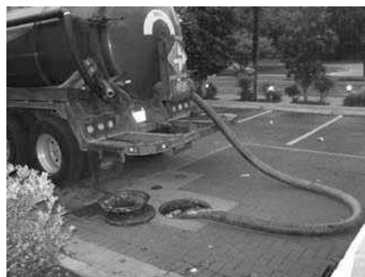
Grease interceptor pump out
