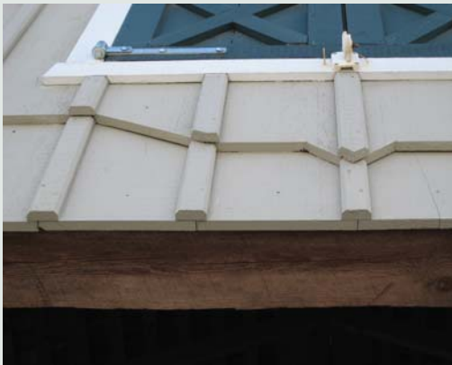
Figure 3.17: Board and Batten Siding Detail at Caves Farm
