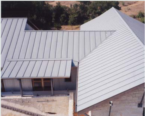
Figure 10.20: Standing Seam Metal Roofing
