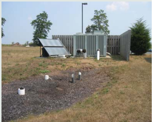
Figure 10.11: Above-Ground Components of a Solar Hot Water System at Adams County Ag Center
