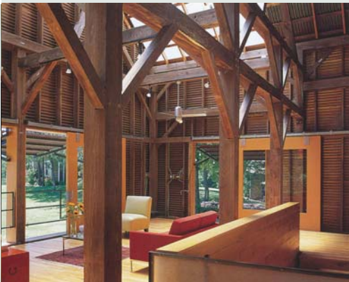
Figure 10.22: Wood Timber Structural Framing
