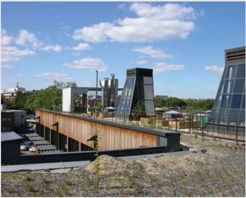
Figure 10.26: Solar Chimneys
