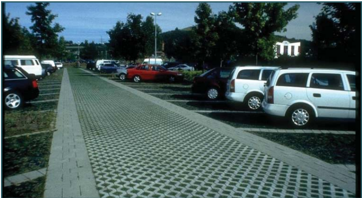
Figure 6.12: Innovative Pervious Paving Materials
