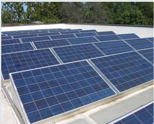
Figure 10.10: Roof-Mounted Array of Photovoltaic Panels
