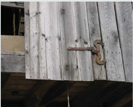
Figure 7.25: Shutter Hinge at Colhoun Farm
