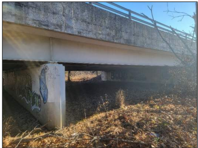
Figure 3: Red Run Boulevard Bridge Clearance
