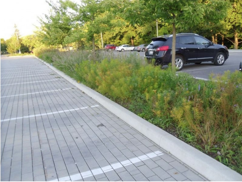
PERVIOUS PAVING USED IN A PARKING LOT
