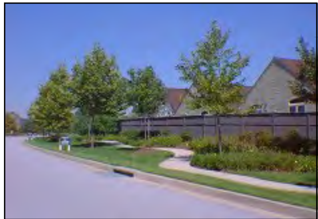
Screening of a dwelling unit is required where its side or rear lot line abuts a public right-of-way.
