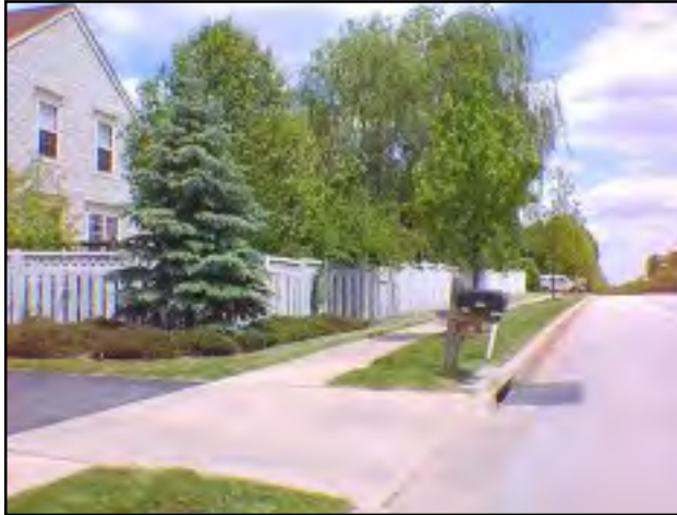
Fencing with plantings on the street side of the fence provides screening where reverse frontage lots are unavoidable.
