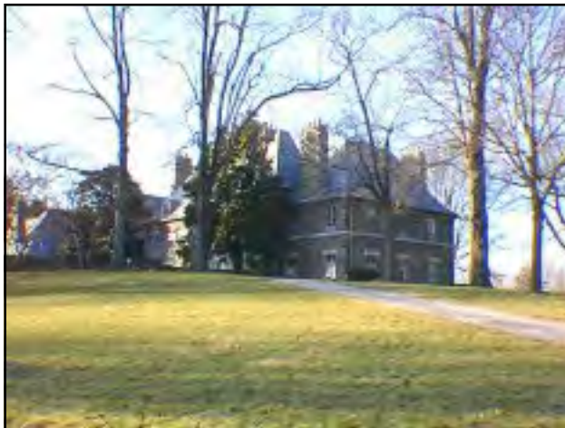
The setting of historic structures should be preserved.
