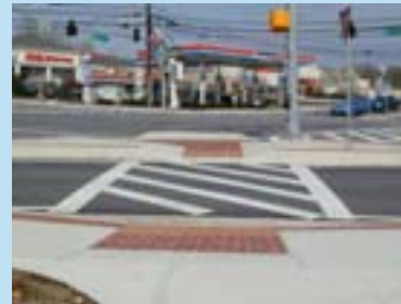
A median offers a pedestrian refuge at the center of a wide street (top, left), paint and stamping is used to dress up a crosswalk (top, right) and, brick pavers are used to accentuate curb ramps (left).
