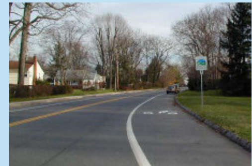
Examples of bicycle lanes: one with a parking lane (top), and one without (middle). When parking needs are few and traffic is light, a parking and bicycle lane can be combined, as was done on Edmondson Avenue (bottom).
