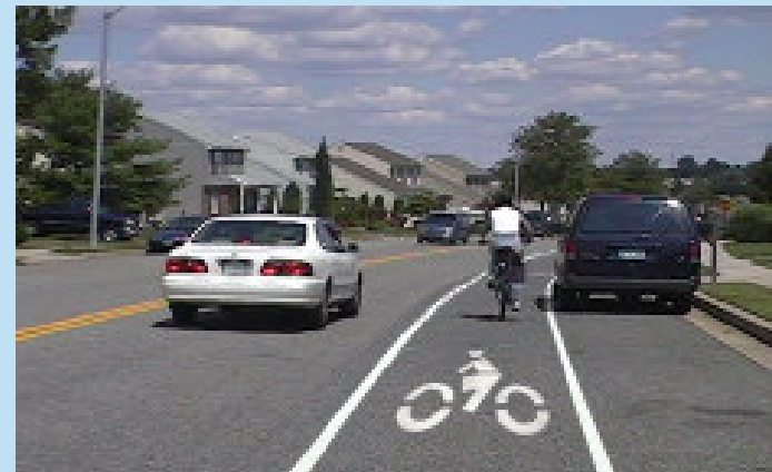
The computer enhanced photograph on the bottom illustrates how bike lanes can be striped on wide roadways. Adding the striping also narrows the area available to motorists, acting as a traffic calming measure.
