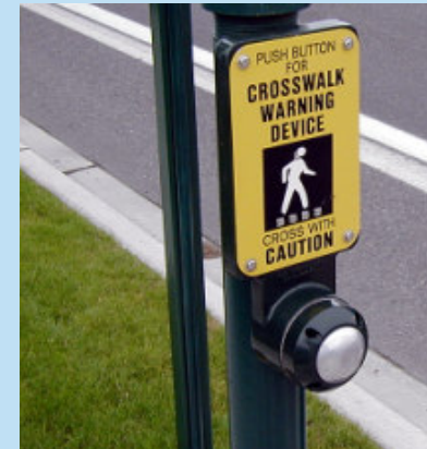
Pedestrian crossing signals count the seconds remaining to cross the street are available (top), as well as push button devices that activate the crossing signal and extend the crossing time (right).
