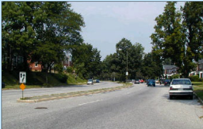
Many of the county's roads are wide enough to accommodate bike lanes by striping or by narrowing the traffic lanes, which are category type 3a and 3b improvements, respectively.
