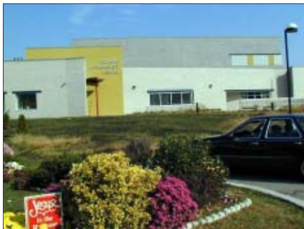
The Fleming Center recreational building was constructed in the 1990's and functions as the hub of the community.
