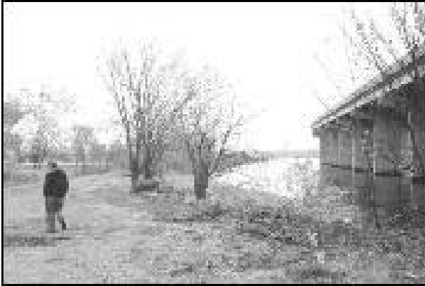
Waterfront reclamation projects are currently underway.
