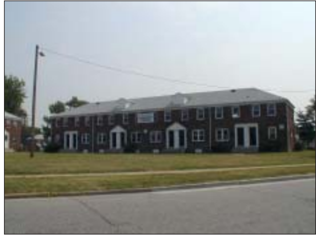
A section of housing in the Day Village community.
