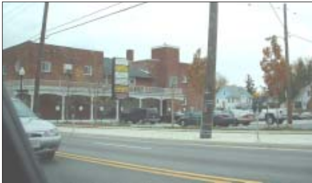
1100 Reisterstown Road may be redeveloped with new retail and office construction.
