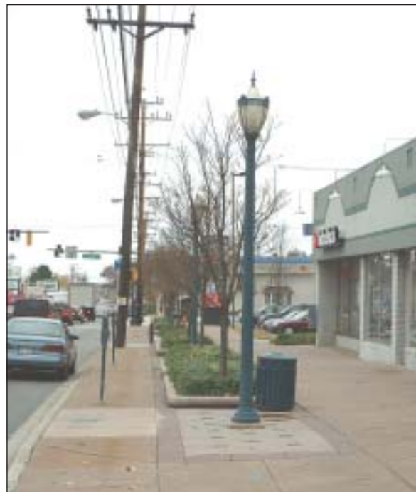
Explore the feasibility of undergrounding or relocating utilities to the rear of businesses.
