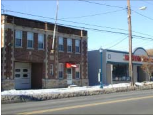
Pikesville Firehouse has the potential to be redeveloped as a restaurant.
