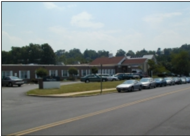
Nursing home at 111 West Road
