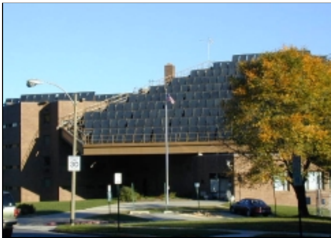
Existing detention center
