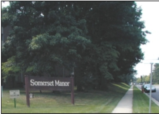
Somerset Manor Apartments
