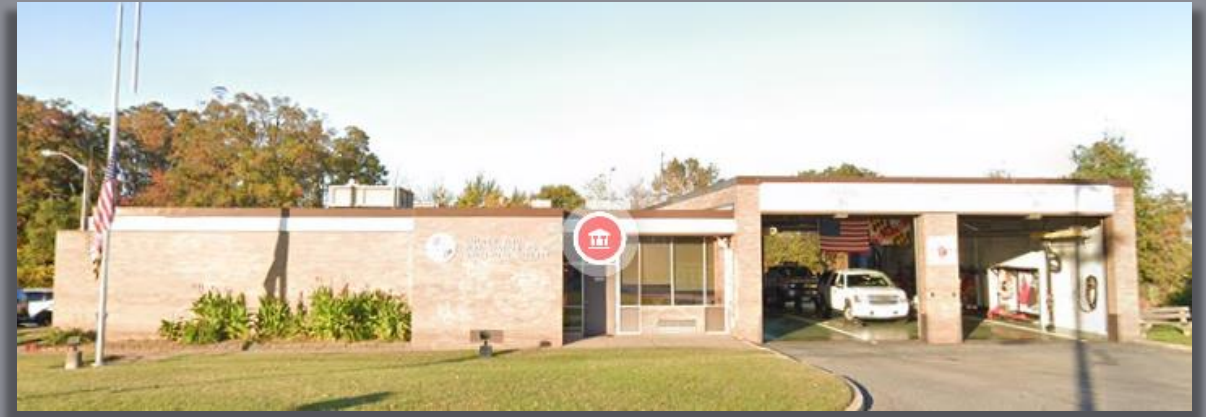
GOLDEN RING FIRE Replace HVAC system
